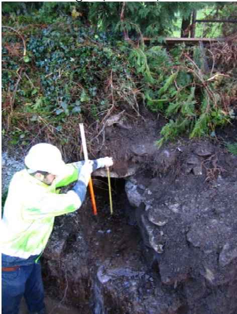
Plate 43: Box culvert along L3402 local road.
