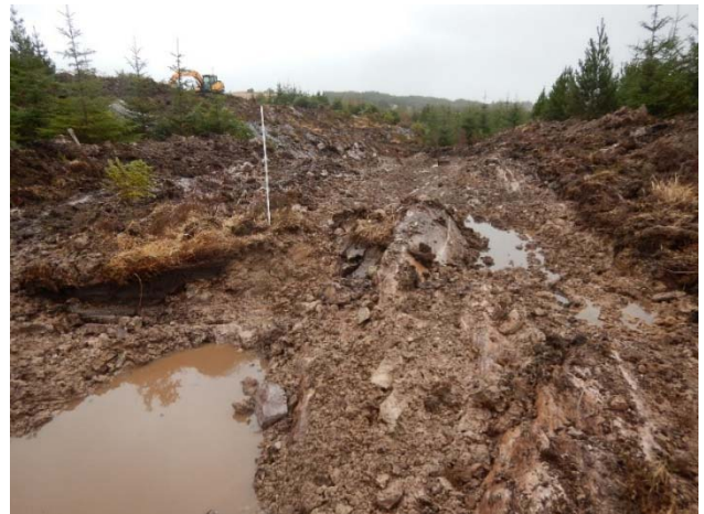
Plate 15: T5 after scrub and peat removal showing natural gravel and rock.
