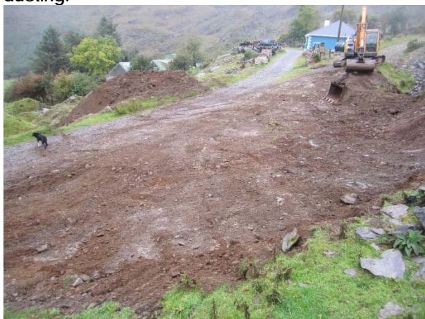
Plate 35: Removal of topsoil at southern end of off-road section of the cable route.
