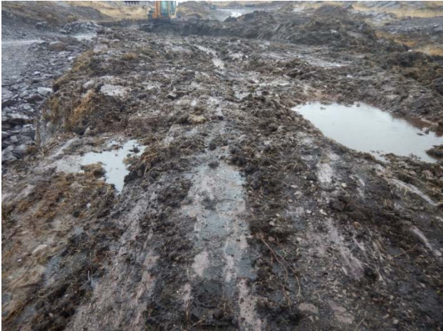
Plate 5: Removal of peat at T9 revealing natural rock and pockets of peat.
