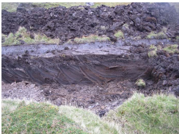
Plate 33: Removal of peat in advance of cable ducting, peat measured 1m (maximum)
