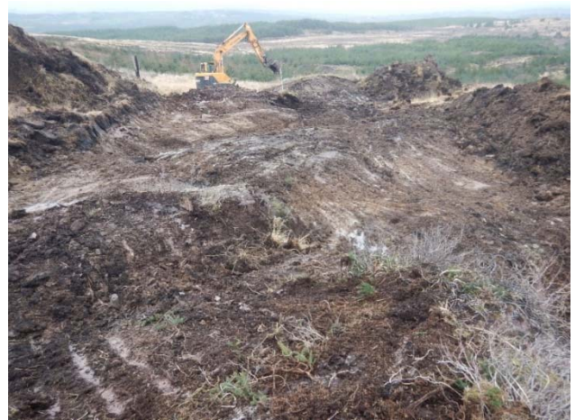
Plate 14: Continuation of road between T8 and T5 after scrub was removed and prior to rock breaking.
