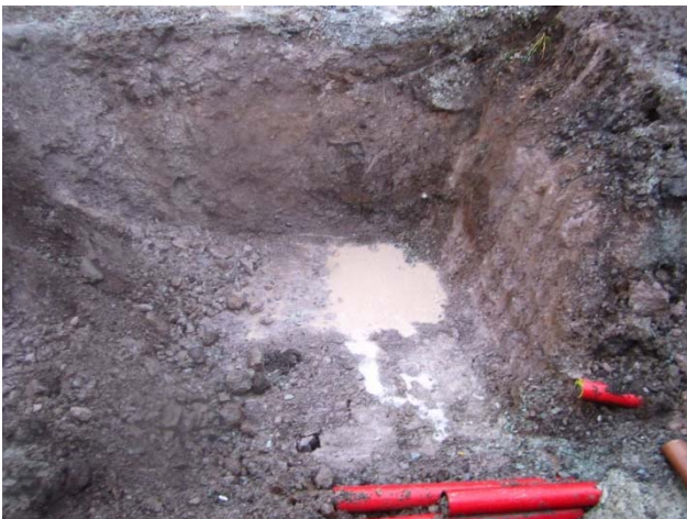
Plate 44: Joint bay along the L3402
