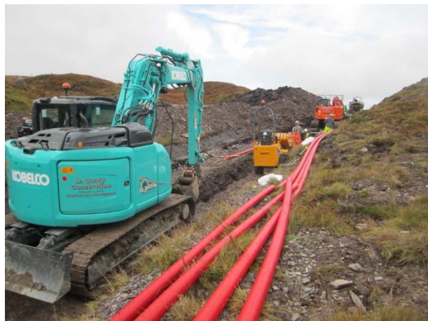
Plate 36: Cable ducting along off-road section of cable route along previously topsoil stripped areas.
