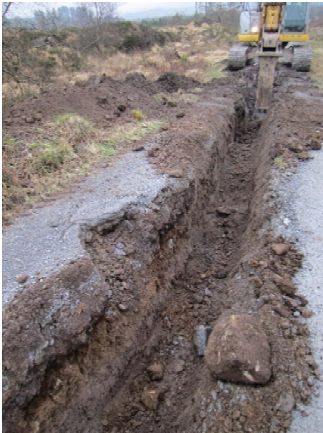
Plate 51: Ducting on road to west of Cleanrath windfarm.
