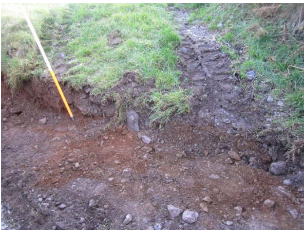
Plate 39: Topsoil removal at road margin in advance of ducting at Gurteenowen townland (ITM E513024 N569567).
