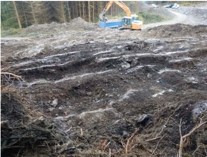
Plate 29: Northern access road during monitoring ridges of natural rock under shallow peat.
