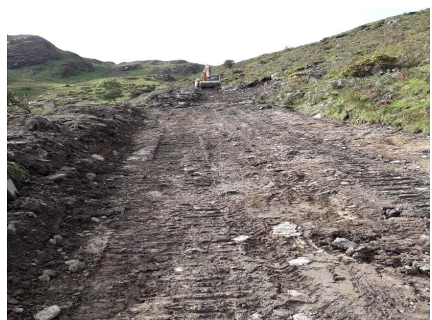
Plate 32: Clearance of cable route in advance of trench excavation.
