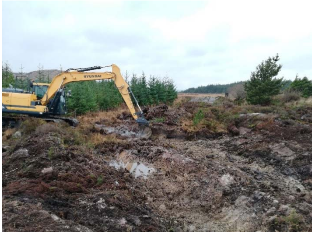
Plate 22: Removal of heather and tree stumps at road leading to T1 looking West
