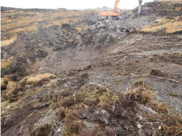
Plate 11: Removal of scrub overlying rock along access road between T8 and T5.
