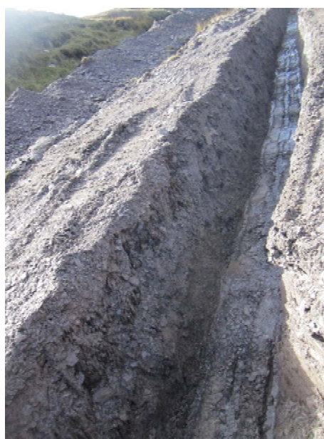
Plate 37: Cable trench 1.2m in depth excavated through natural soil.
