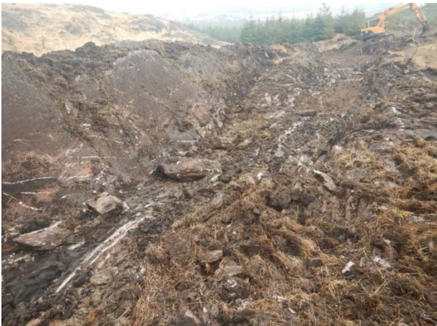
Plate 13: Shallow peat removal in area of T8, numerous rock outcrops visible.
