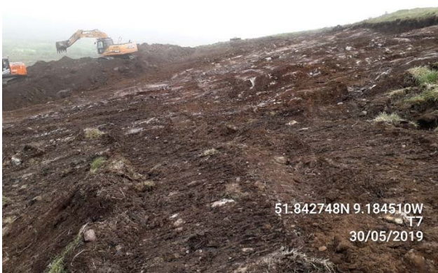
Plate 2: T6 after clearance of peat, revealing natural rock.
