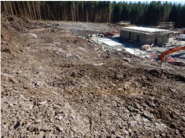
Plate 25: Substation site after site clearance and peat removal.
