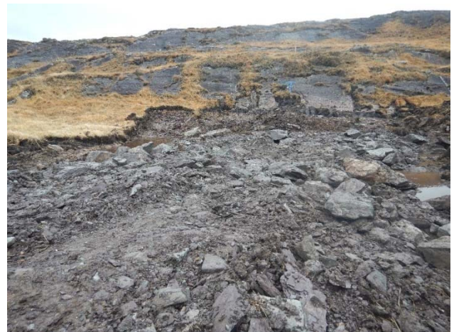
Plate 9: T10 turbine hardstand, shallow peat over natural rock.
