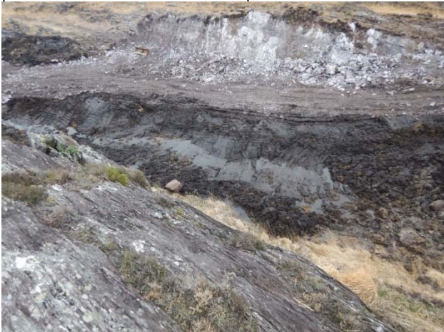
Plate 6: Peat removal along access road from T9 to T8 in between two rocky outcrops.
