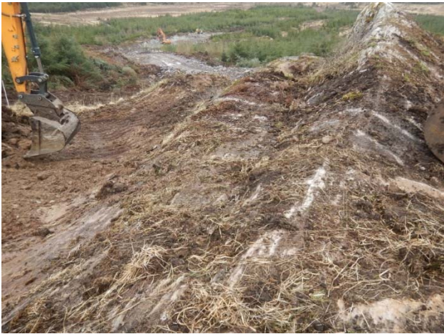
Plate 12: Monitoring removal of scrub and shallow peat over rocky veins between T10 and T8 access road.
