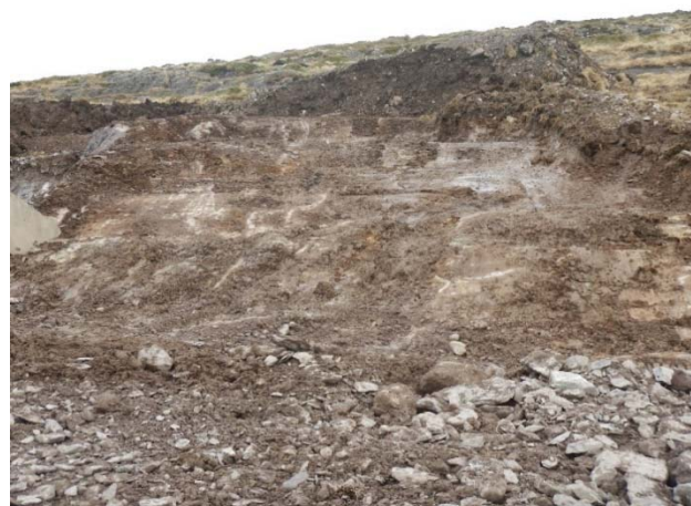
Plate 4: removal of shallow peat over natural rock outcrop.
