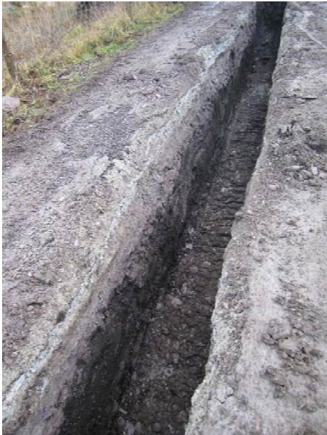
Plate 48: Ducting showing peat below road make-up.
