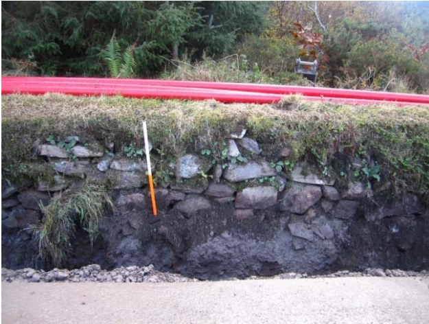
Plate 42: Continuation of cabling along the L3402. Road-side stone wall exposed and remained in situ.
