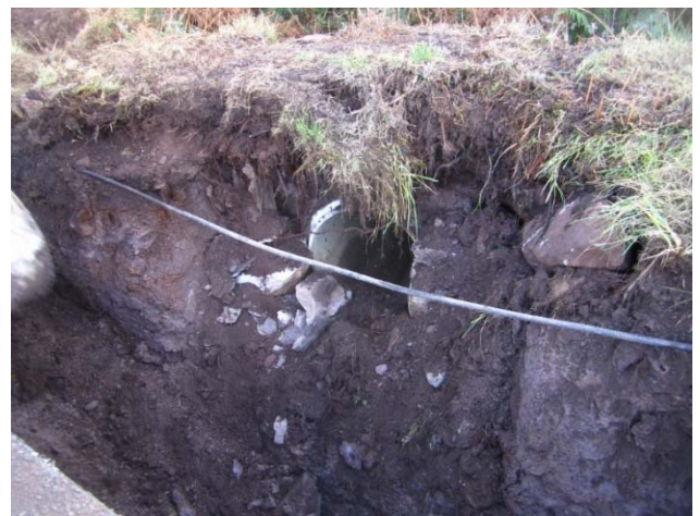
Plate 41: Modern culvert crossing cable trench.
